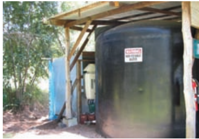
Figure 10.6 —Black water storage tanks are a low-cost way to warm irrigation water with solar energy before it is applied to crops. Photo by Thomas D. Landis.
